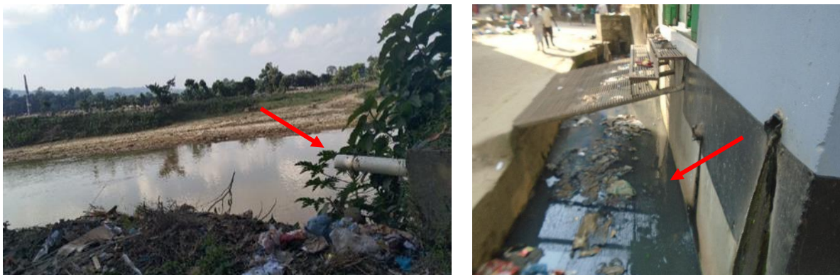
Figure 6: Containment technologies and their connections in Khagrachari. Left: Toilet Pit open to a nearby water body, Right: Toilet pipe connected to open environment. (Source: Feasibility study 2020-21/DPHE).
