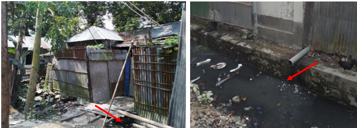
Figure 6: Containment technologies and their connections in Kurigram. Left: Toilet Pit open to a nearby water body, Right: Toilet pipe connected to open environment. (Source: Feasibility study 2020-21/DPHE ).
