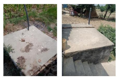
Figure 3: Fully lined tank built near the farmland in household level.
