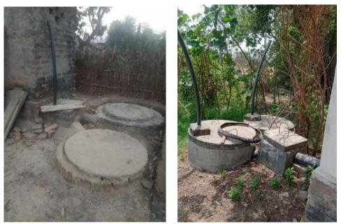
Figure 5: Twin pits with proper distance as seen in household.
