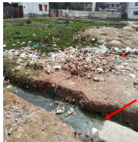
Figure 6: Containment technologies and their connections in Kushtia. Left: Toilet Pit open to a nearby water body, Right: Toilet pipe connected to open environment. (Source: Feasibility study 2020-21/DPHE ).
