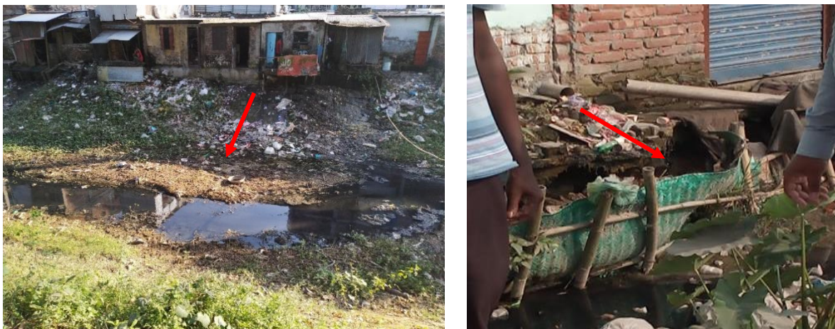
Figure 6: Containment technologies and their connections in Manikganj. Left: Toilet Pit open to a nearby water body, Right: Toilet pipe connected to open environment. (Source: Feasibility study 2020-21/DPHE).
