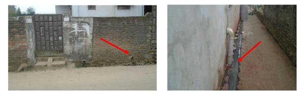
Figure 6: Containment technologies and their connections in Mymensingh. Left: Toilet Pit open to a nearby water body, Right: Toilet pipe connected to open environment. (Source: *Feasibility study 2020-21/DPHE*).
