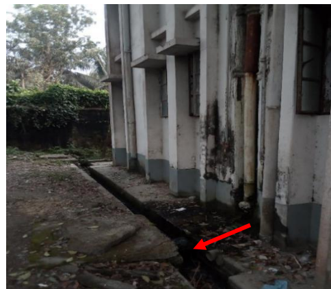
Figure 6: Containment technologies and their connections in Madaripur. Left: Toilet Pit open to a nearby open environment, Right: Toilet pipe connected to nearby drain. (Source: Feasibility study 2020-21/DPHE ).
