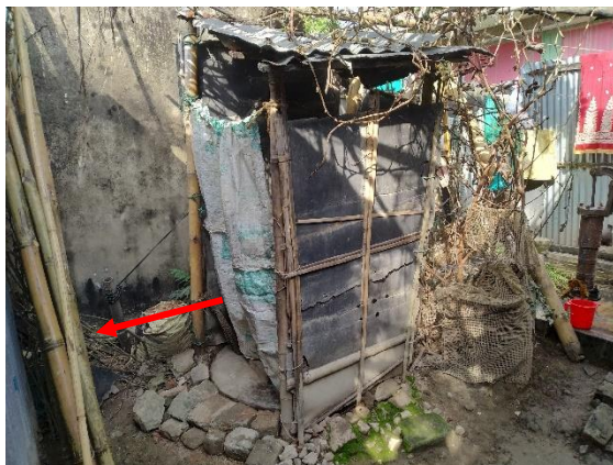
Figure 6: Containment technologies and their connections in Madaripur. Left: Toilet Pit open to a nearby open environment, Right: Toilet pipe connected to nearby drain. (Source: Feasibility study 2020-21/DPHE ).
