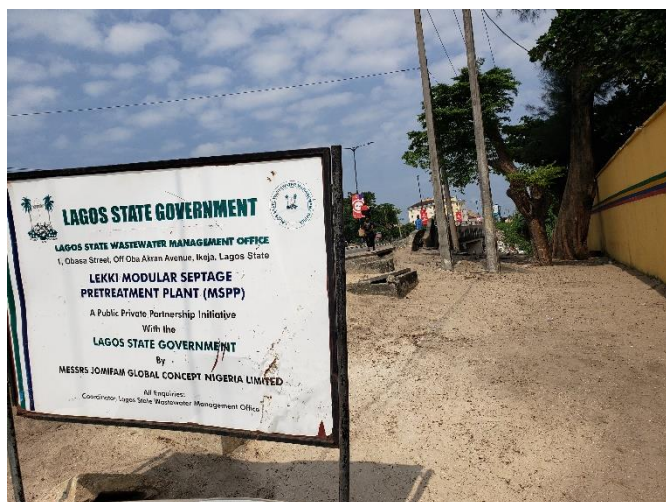
Fig 7 Modular Septage Treatment Plant in Lekki
