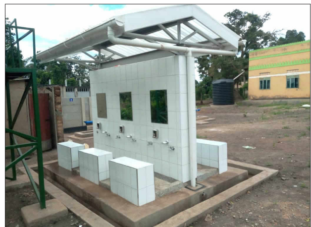
Above: Design of an ablution station constructed at Sanitation for Millions beneficiary mosques.
