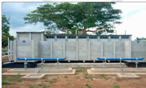
Above: Gender segregated dry-lined toilet facility constructed at a church in Apac Municipal Council
