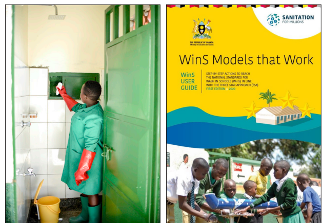
Left: Emptying of the used sanitary towels into to the incinerator connected to the Menstrual Hygiene change room on the model toilet facility; Right: The WASH in Schools - Models That Work publication.
