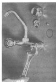
3-Remove the internal part of valve by using appropriate wrench
