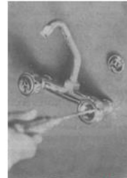
2-Remove screw by using appropriate screwdriver
