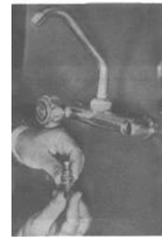
4-Replace old rubber ring inside faucet and reinstall all parts
