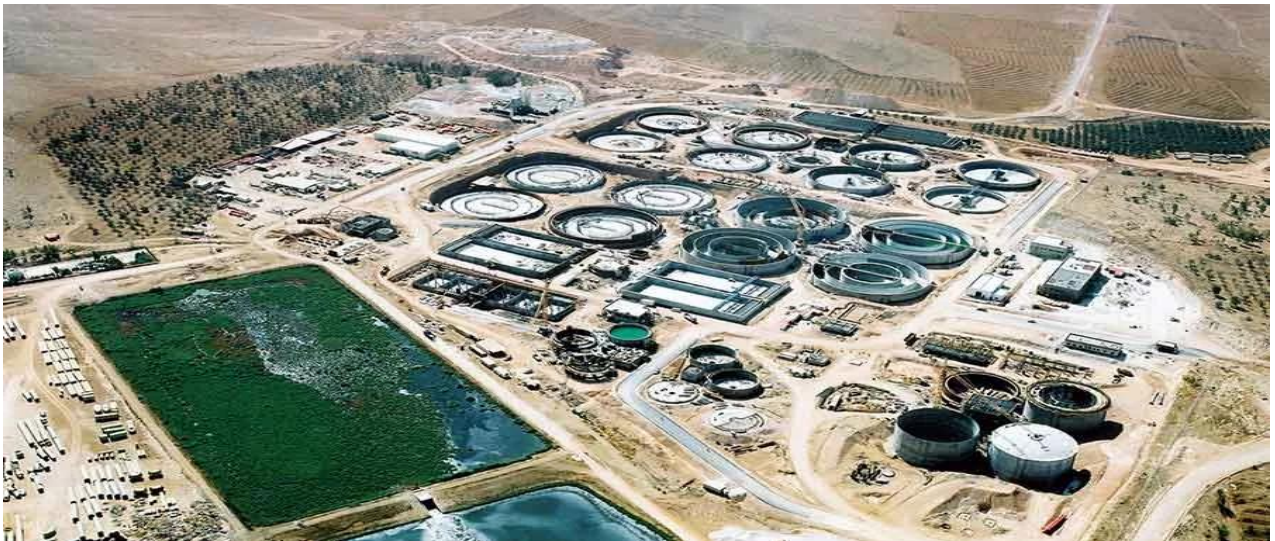
Figure 1: Asamra WWTP – the largest WWTP in Jordan
