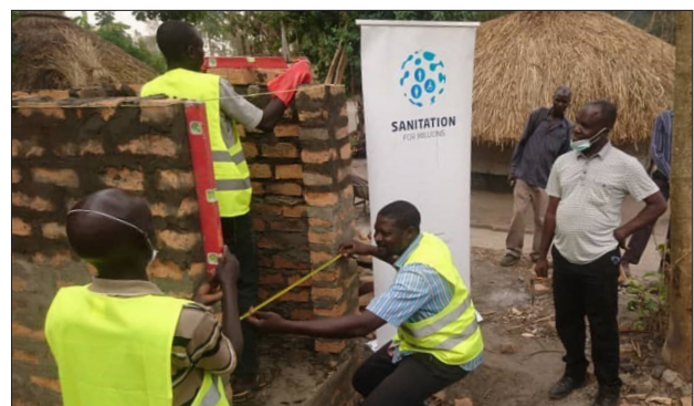
Above: Toilet construction demonstrative session at a Household in Apac.
