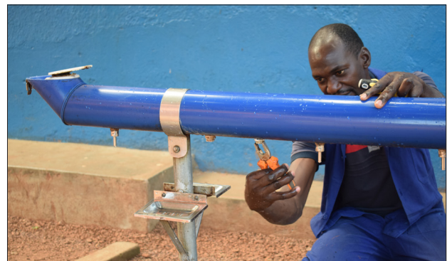
Above: A trained Hausmeister fixing a broken nozzle on the WASHaLOT handwash station.
