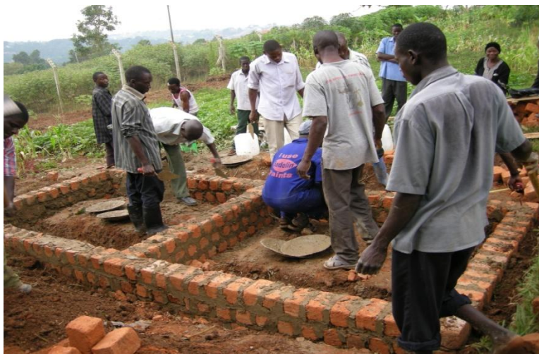
Training of masons in UDDT construction, Mukono, Uganda
