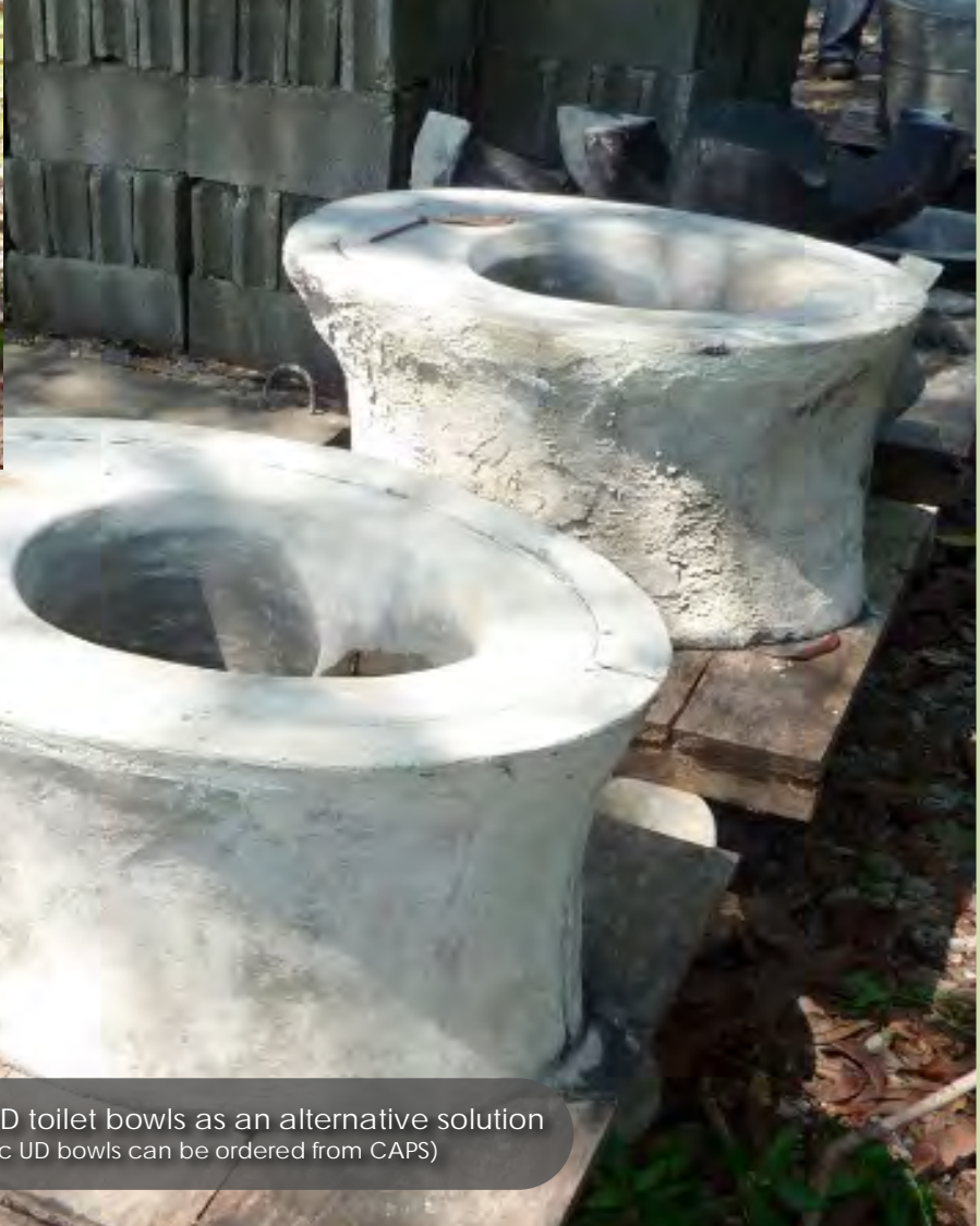
1 production of simple concrete arborloo bowls
