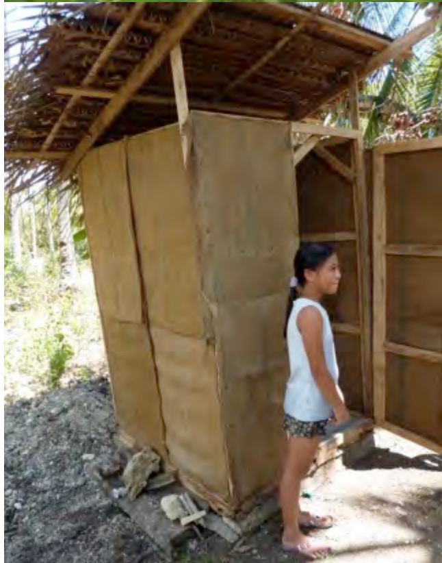
Interior of the arborloo (concrete floor, container for covering material & EcoPee urinal)
