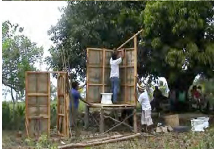
5 setting up of walls
