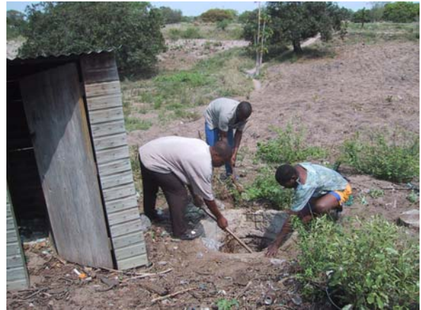
The site on inspection in 2003. The 200 litre drum in the toilet was full. The 1m diameter concrete lined pit was half full.
