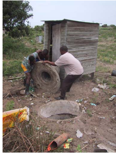
The ring lined pit with 2 bags of leaves at the base. Rolling the concrete slab over onto the newly excavated pit.
