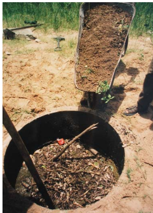
Humus like soil being added to used pit (2000)
