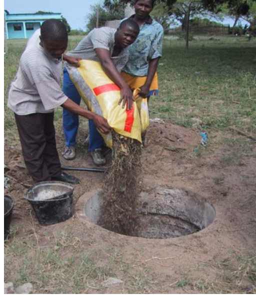
Two full bags of dried leaves were thrown down the pit. These leaves help to start the conversion process from excreta into humus. The family members are encouraged to put down soil regularly into the pit and also leaves. They are also encouraged not to put down rags and other garbage.
