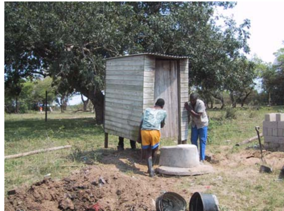
The slab and pedestal are placed on the newly emptied pit. This is followed by placing the superstructure over the pit.
