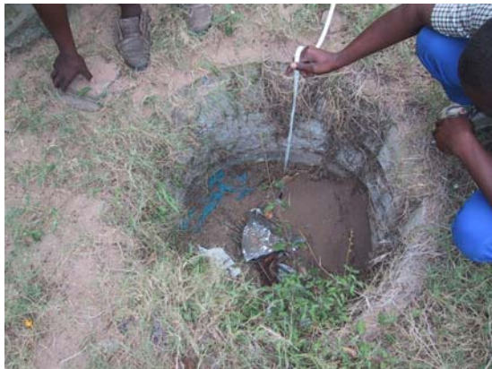
On the left the pit as it was found with a soil like surface. Most of the pit contents were humus like and relatively easy to dig out. There were many rags and bits of wood. Three men took turns to dig out the remaining 1meter of contents which took one hour.
