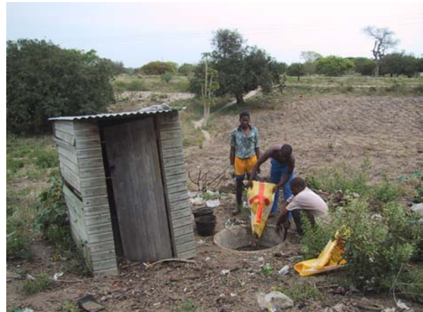
Plastic bags were used as gloves on this experimental excavation. Protective clothing for this job is important. Once emptied, two full bags of dried leaves were added to the 2m deep pit.
