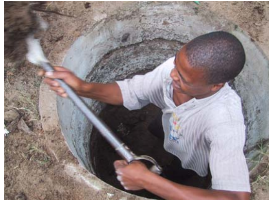
On the left the pit as it was found with a soil like surface. Most of the pit contents were humus like and relatively easy to dig out. There were many rags and bits of wood. Three men took turns to dig out the remaining 1meter of contents which took one hour.
