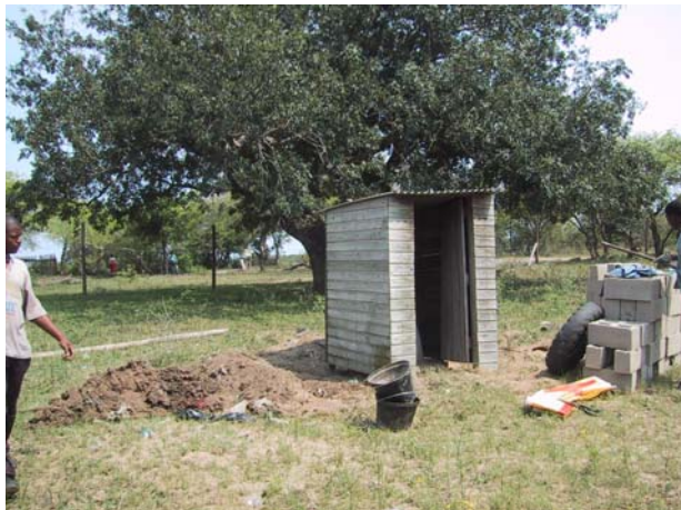
Finally the site is cleared and prepared for use. The family are requested to add leaves and soil to the pit regularly. In this case 5 litres of soil per week. Leaves should also be added from time to time. The pit will be examined in the future to test the filling rate (16 persons). The whole job was completed in 2 hrs.
