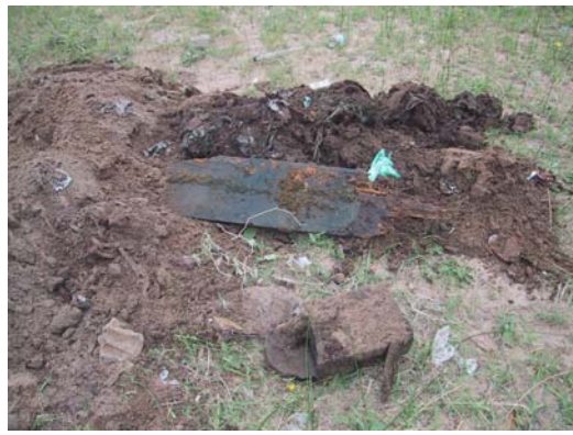
The pit being emptied. The men wore plastic gloves made of old bags. A pile of excavated pit contents was built up around the pit. Note the wood and other rubbish.
