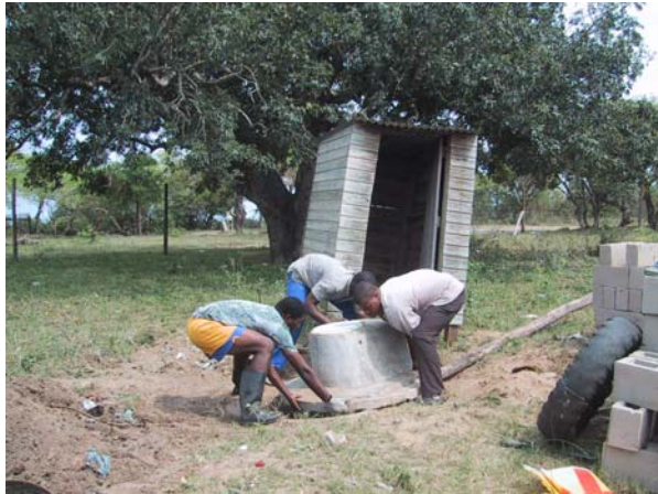
The slab and pedestal are placed on the newly emptied pit. This is followed by placing the superstructure over the pit.
