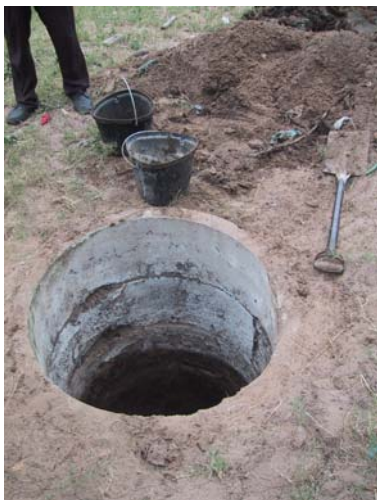
On the left the completed excavation leaving a pit 2m deep and 1m in diameter. On the right the men gather dried leaves. These will be placed down the pit.
