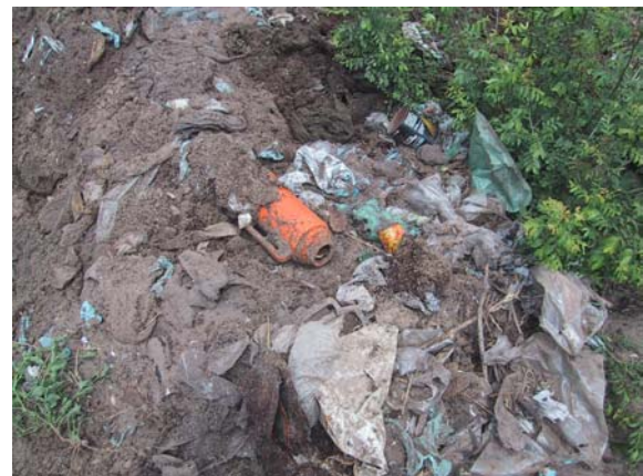
Buckets were used in rotation to take out the pit contents. The short spade also helped. A great deal of rubbish, mostly plastic and rags was also excavated.
