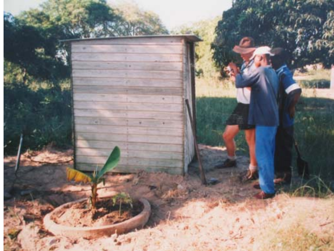
The toilet as it was left in 2000 with trees planted on the pit covered with soil
