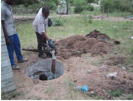
The pit being emptied. The men wore plastic gloves made of old bags. A pile of excavated pit contents was built up around the pit. Note the wood and other rubbish.
