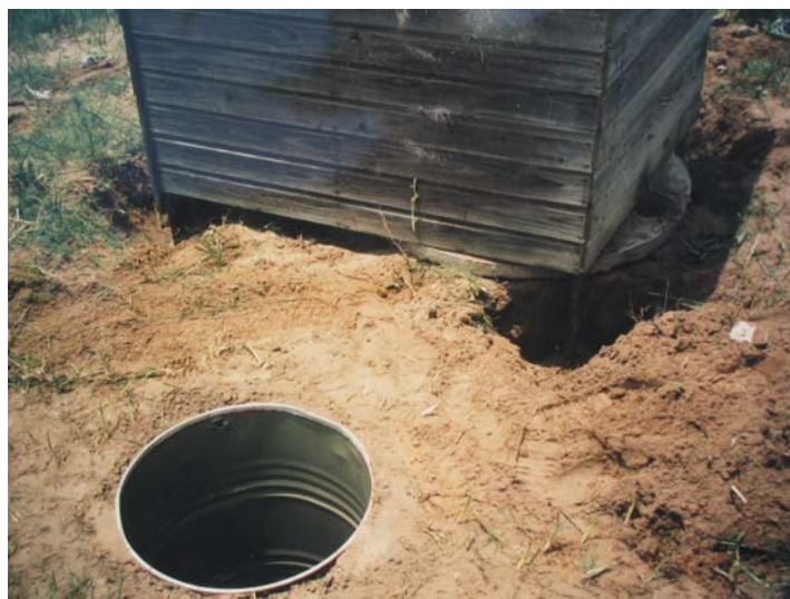
The 200 litre drum dug into the sand next to VIP latrine
