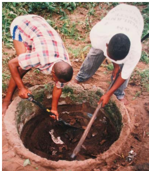
Digging out the top of pit filled 8 years earlier
