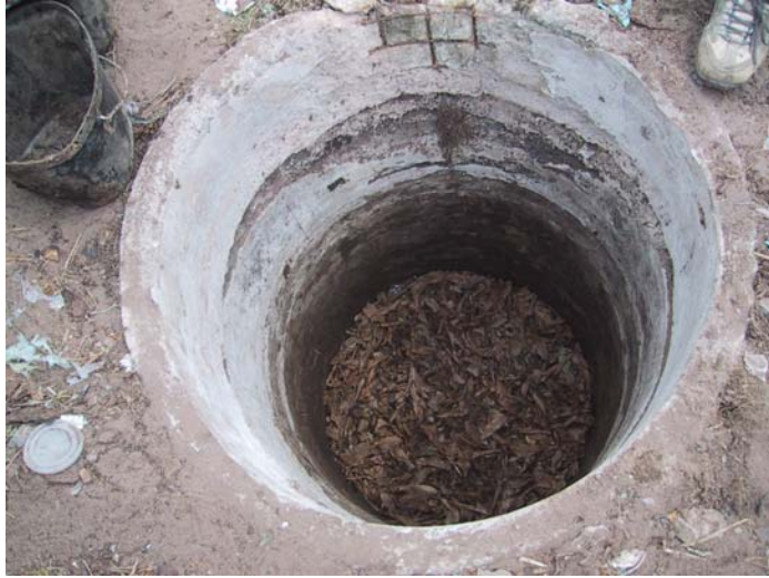
The ring lined pit with 2 bags of leaves at the base. Rolling the concrete slab over onto the newly excavated pit.
