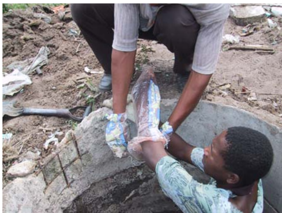
Plastic bags were used as gloves on this experimental excavation. Protective clothing for this job is important. Once emptied, two full bags of dried leaves were added to the 2m deep pit.
