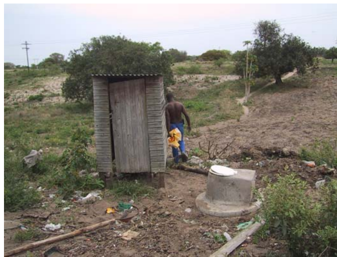
The site as it was left with slab and pedestal over newly excavated pit.
