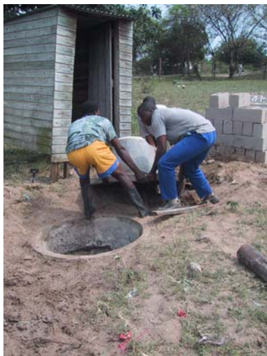
The concrete slab is moved from the drum pit to the larger pit. The drum is filled with soil
