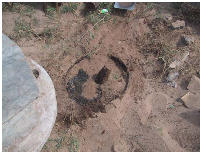
The concrete slab is moved from the drum pit to the larger pit. The drum is filled with soil
