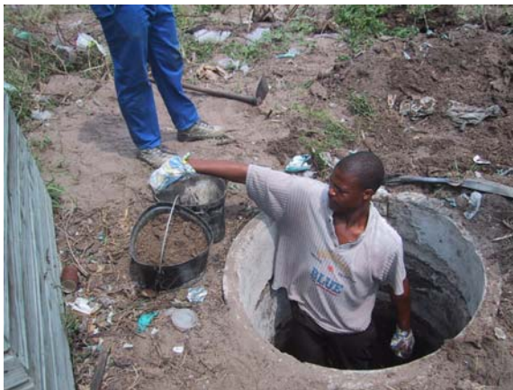
Buckets were used in rotation to take out the pit contents. The short spade also helped. A great deal of rubbish, mostly plastic and rags was also excavated.
