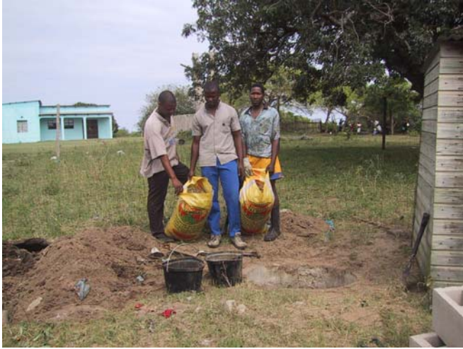
Two full bags of dried leaves were thrown down the pit. These leaves help to start the conversion process from excreta into humus. The family members are encouraged to put down soil regularly into the pit and also leaves. They are also encouraged not to put down rags and other garbage.
