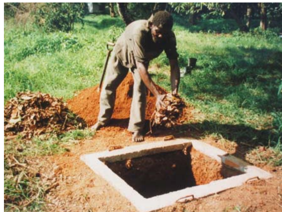
Adding semi composted palm leaves to the base of a Fossa alterna pit in Mombasa, Kenya (left). Adding leaves to a Fossa alterna pit at Fambidzanai, the Permaculture Association of Zimbabwe.
