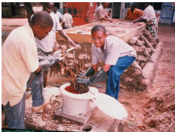
Adding semi composted palm leaves to the base of a Fossa alterna pit in Mombasa, Kenya (left). Adding leaves to a Fossa alterna pit at Fambidzanai, the Permaculture Association of Zimbabwe.
