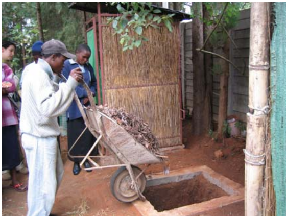
Adding leaves to Fossa alterna pits. On left at Woodhall road, on right at Epworth, near Harare.
