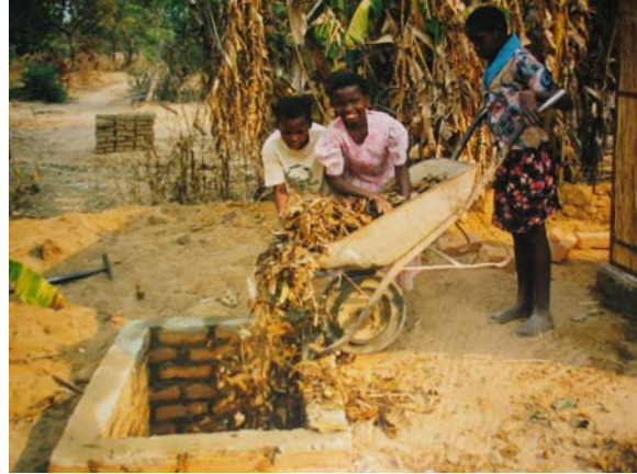
Adding leaves to Fossa alterna pits. On left at Woodhall road, on right at Epworth, near Harare.
