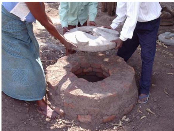
Installing small slab on bring ring beam for Arborloo
