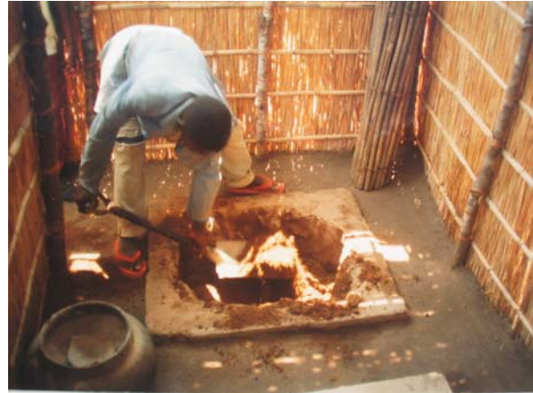
Digging out the compost from Fossa alterna, Mozambique.
