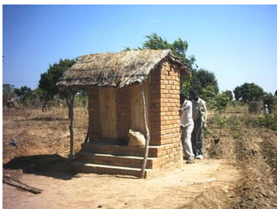
Urine diverting toilet in CCAP project Malawi
