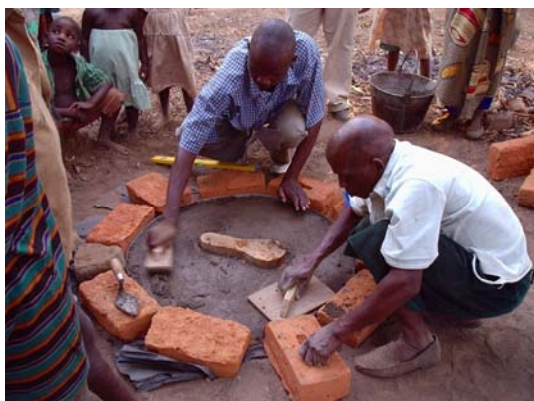
Making concrete slab for eco-toilets. Malawi
