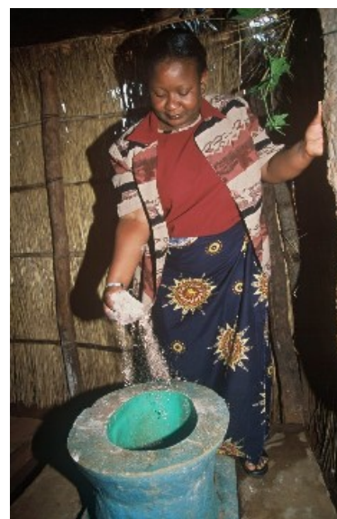
Adding ash to a Fossa alternata in Lichinga, Mozambique. WaterAid UK.
