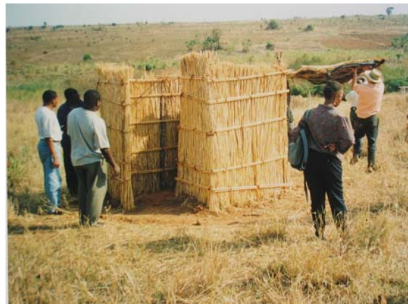
Grass structure being built in Lichinga, Mozambique
