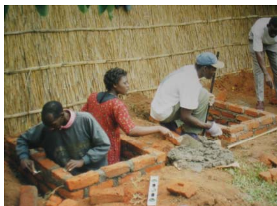
Training in making brick ring beams. WaterAid. Lilongwe
