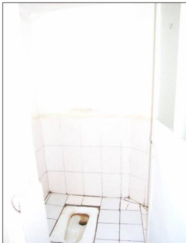
Pic. 5: A pour-flush toilet of a newly constructed house (source: N. Khawaja).
