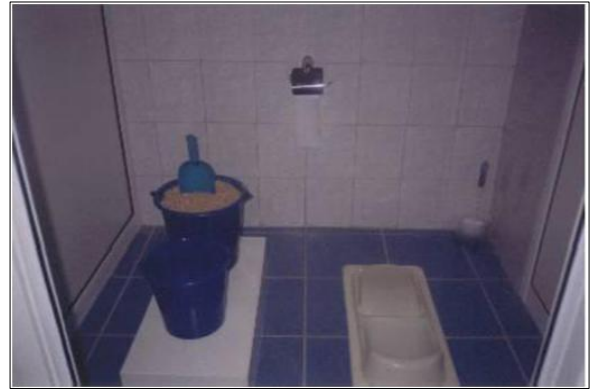
Pic. 9: A double vault UDDT in a school in Hayanist, Armenia showing one squatting pan out of use and covered with a lid and a bucket of sawdust and one squatting pan in use (source: Deegener et al., 2009).
