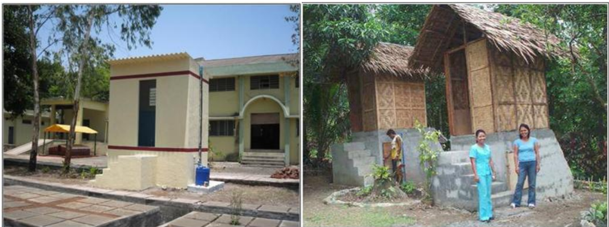
Pic. 10 - 11: A double vault UDDT in India (Left, source: ESF India) and in Sinalac School, Philippines. (Right, source: Sayre & Muench, 2009)
