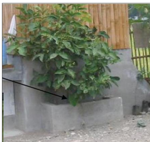
Pic. 18: An evapo-transpiration box at the side of the UDDT (source GTZ, Philippines).
