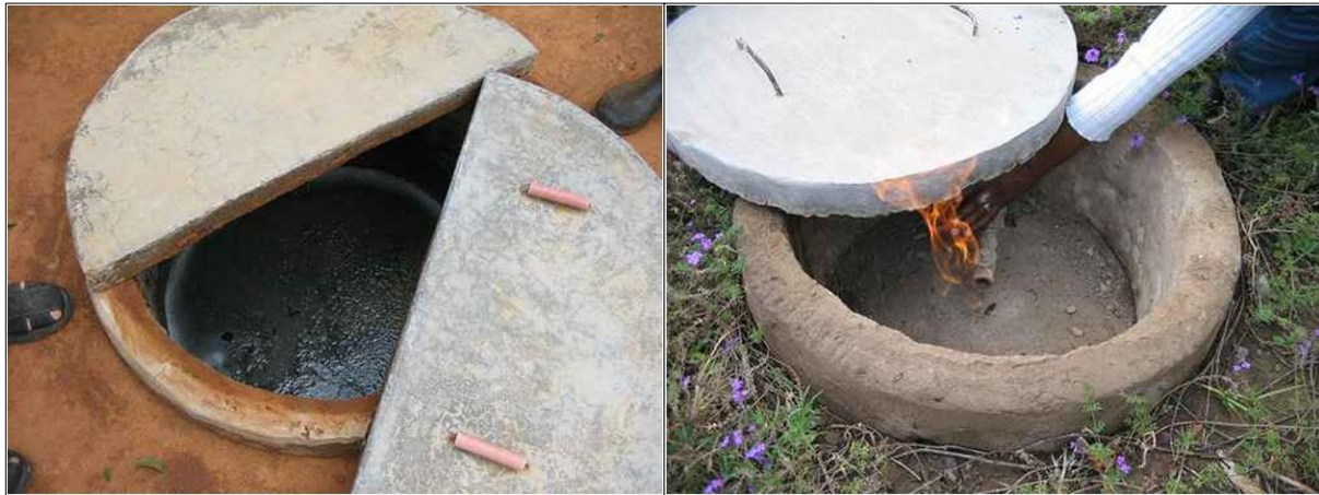
Pic. 25 - 26: Left. Access hole to a biogas digester. Right. Flaring biogas (source: GTZ).
