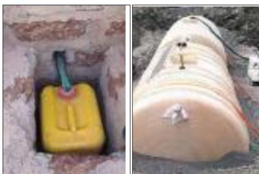
Pic. 16 - 17: Left. A 20 l plastic jerrycan for urine collection (source: E. v. Muench, 2006). Right. A below-ground plastic urine storage tank (source: Kvarnström et al., 2006).
