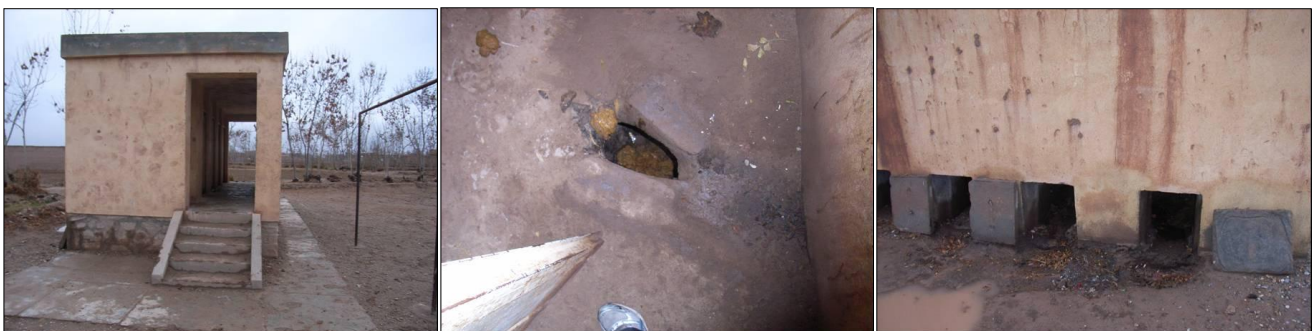
Pic. 6 - 8: The toilet block of the school with 'simple latrines' and opening at the back of the rased vault to remove the excreta (source: N. Khawaja).
