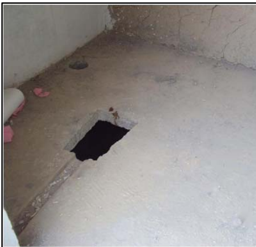
Pic. 9: A moulded concrete slab of a single-vault UDDT with a urine-diverting channel (source: UPDP).
