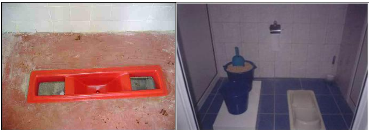
Pic. 5 - 6: Left. A single plastic squatting pan for a double-vault UDDT, with two holes for faeces collection and one hole for urine collection (source: GTZ). Right. A double-vault UDDT in a school in Armenia showing one plastic squatting pan out of use and covered with a lid and a bucket of sawdust and one pan in use (source: Deegener et al., 2009).
