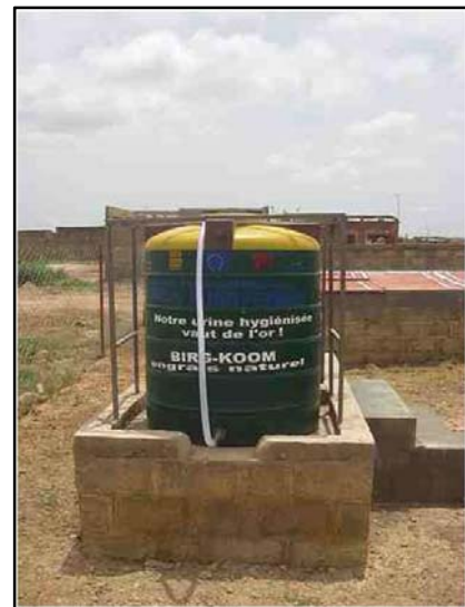
Pic. 16: A urine storage tank in Burkina Faso (source: GTZ).
