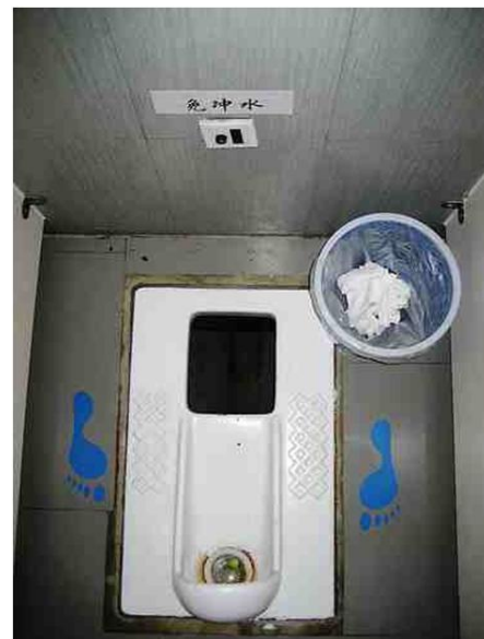
Pic. 20: A urine-diverting squatting pan in a public toilet in China showing the direction of sitting with foot marks (source: GTZ).
