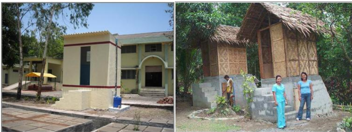
Pic. 3 - 4: A double-vault UDDT in India ( Left , source: ESF India) and in Sinalac School, Philippines ( Right , source: Sayre & Muench, 2009).
