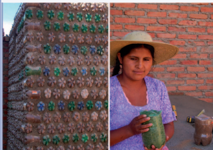
Figure 4: Single chamber toilet built with recycled PET bottles
