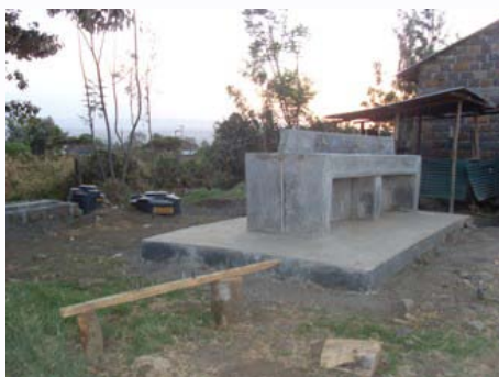
Figure 7: Washing facility- Crater View Secondary School
