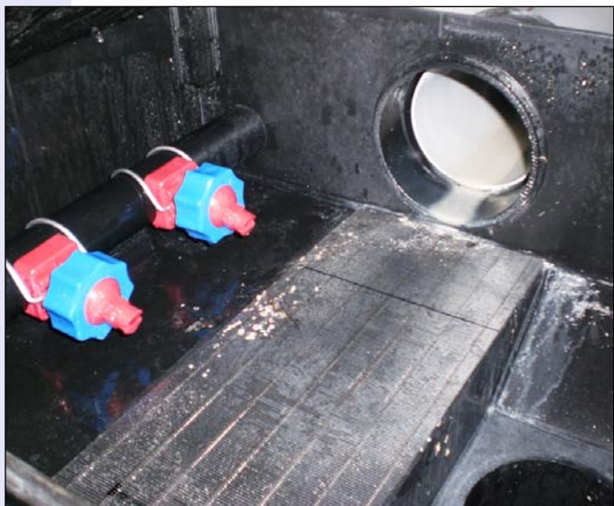
Figure 2: The GEP- TridentMAX, a screen with an mesh size of 0.35 mm separating the raw greywater from the solid ingredients
