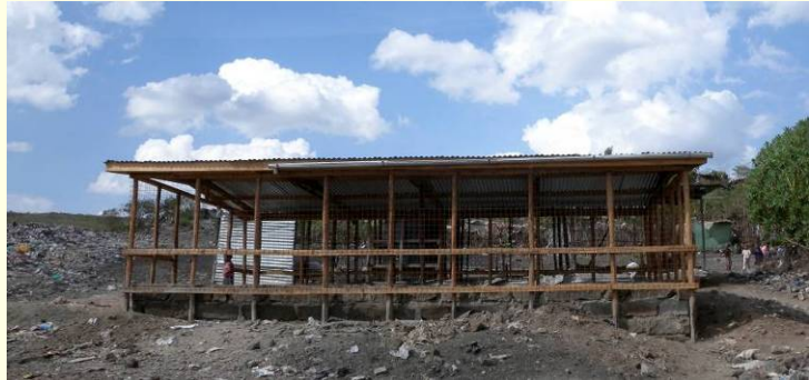
Figure 2: Drying shed at the dump site for centralised composting.
