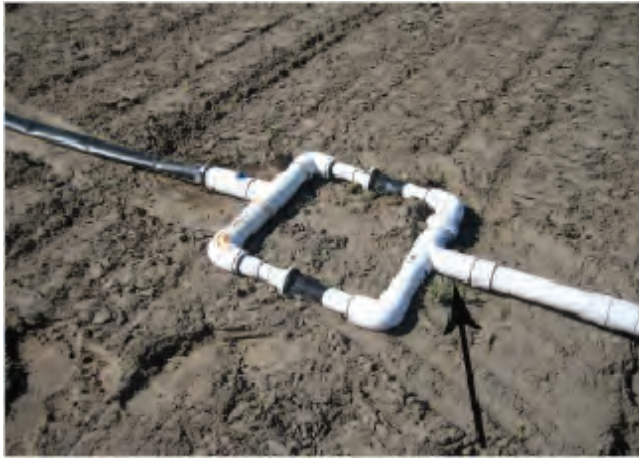
Figure 6. Pressure regulators installed side-by-side allow a greater flow rate.
