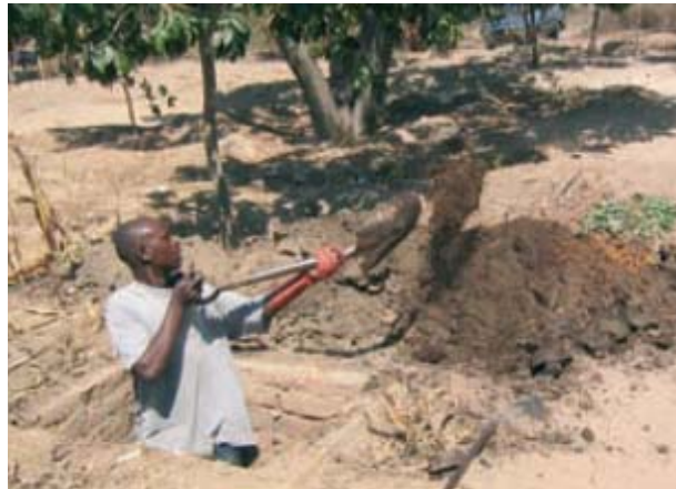
Easy emptying of a dry toilet and a composting toilet.
