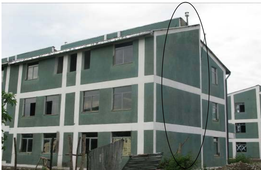
Figure 3: Collection shaft with ventilator at the outside
