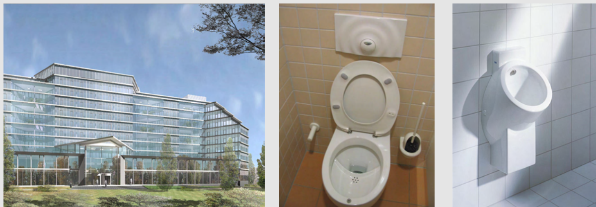
Figure 20: The main building of the GTZ headquarters (left - ttsp-HWP-Seidel); urine diversion toilet (middle - ROEDIGER) and waterless urinal (right; Keramag)
