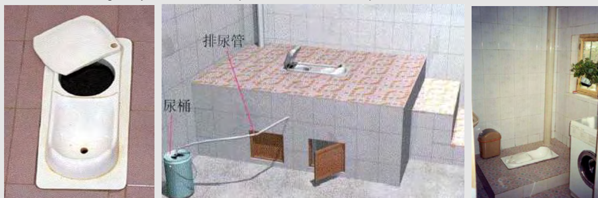
Figure 8: ecosan urine diversion squatting pan (left); ecosan in-house toilets (middle and right) (SIDA)
