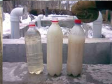
Greywater treatment in Jetygen (from right to left): influent, after pre-treatment, effluent.
