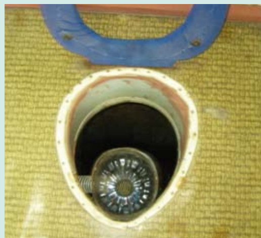
Retro-fitted pit latrine. The funnel for collecting urine is made from a 5-l water bottle.
