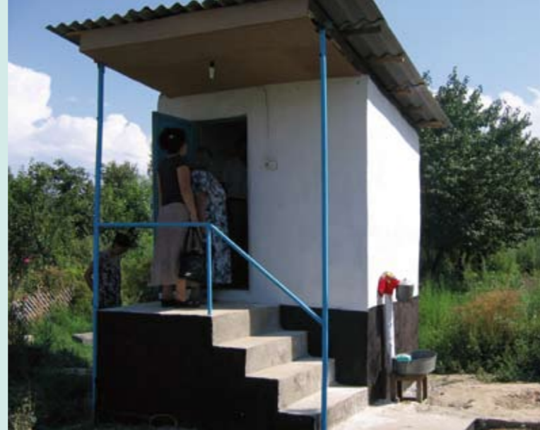
Hygiene is important: note the washstand on the right side of the toilet.
