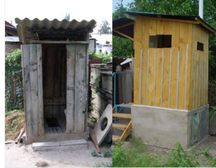
Old and new: pit-latrine (left) and UDDT. Faeces chamber doors are on the right side.
