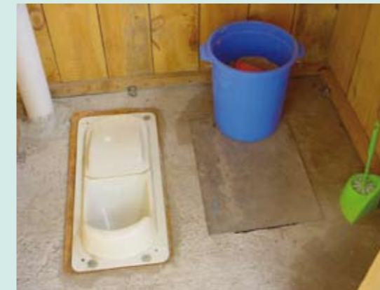
Inside UDDT: the squatting slab is imported from China. The bucket is filled with sawdust for "flushing".
