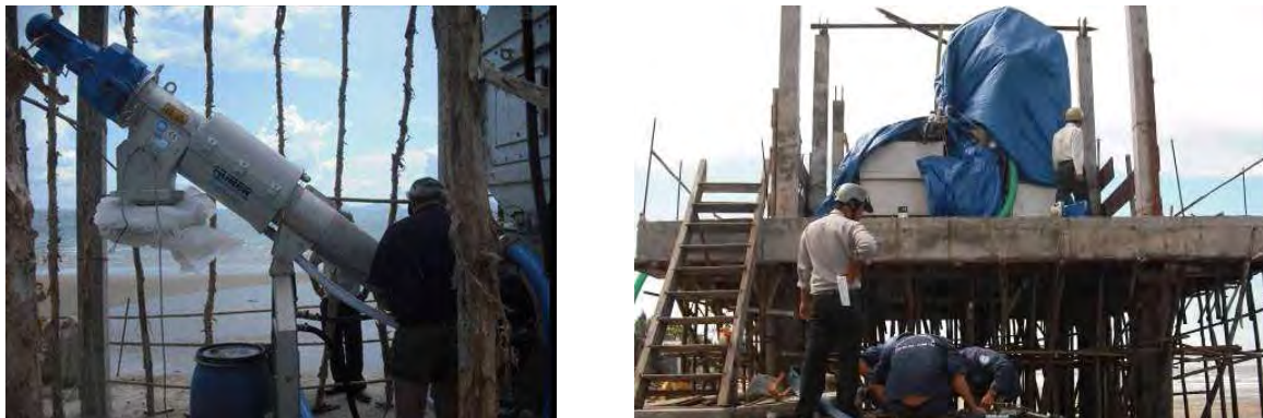
Figure 3: Ultra-fine drum screen (HUBER RoMesh) and screenings compactor (HUBER Ro7) at Long Hai Beach, Vietnam
