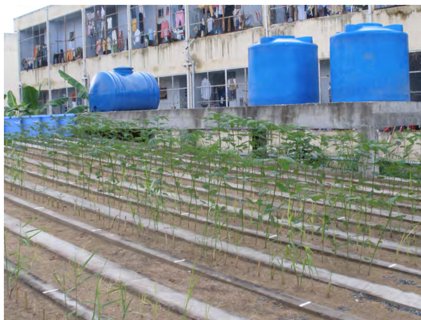
Figure 1: Partial view of the planted soil filter system on the campus of
