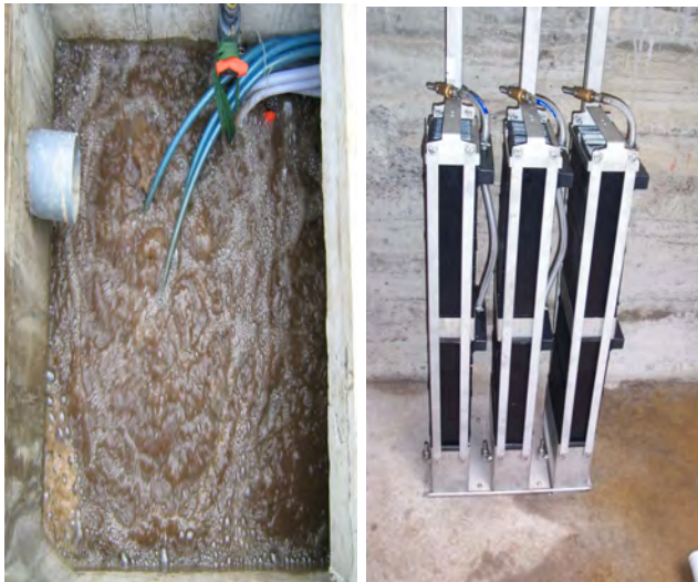
Figure 2: Surface of the activated sludge tank and membrane modules, HUBER GreyUse ® plant
