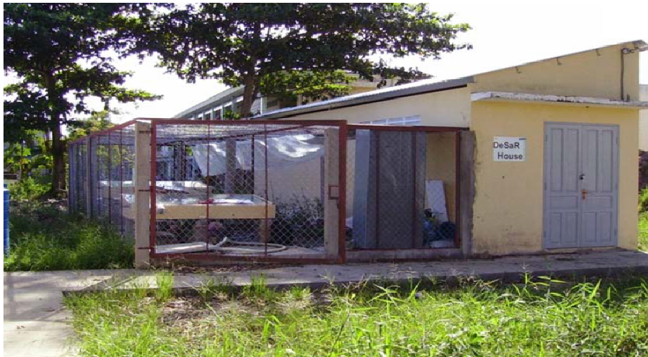
Figure 2: DeSa/R ® House at the Campus of the University in Can Tho
