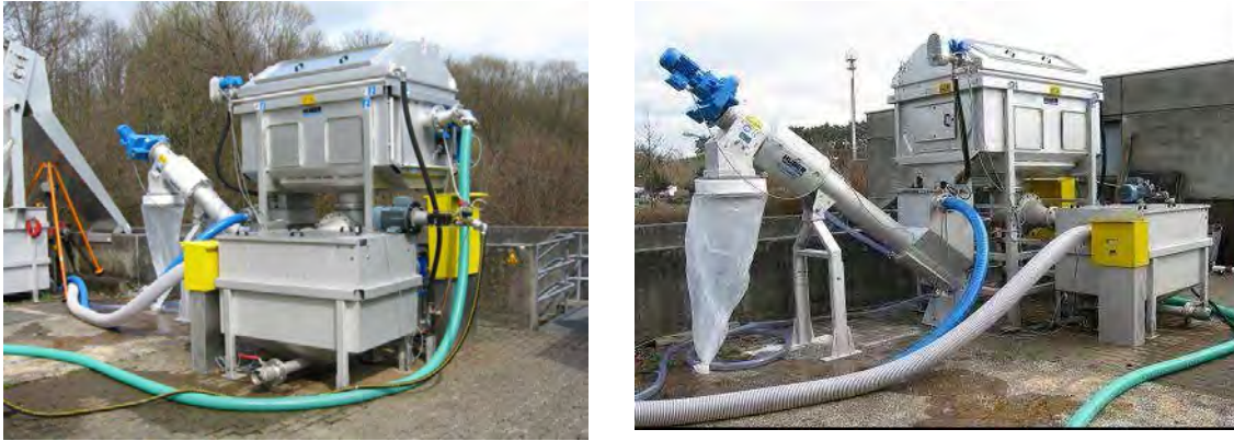
Figure 4: Ultra-fine drum screen (HUBER RoMesh) and screenings compactor (HUBER Ro7) at the WWTP Neumarkt, Germany
