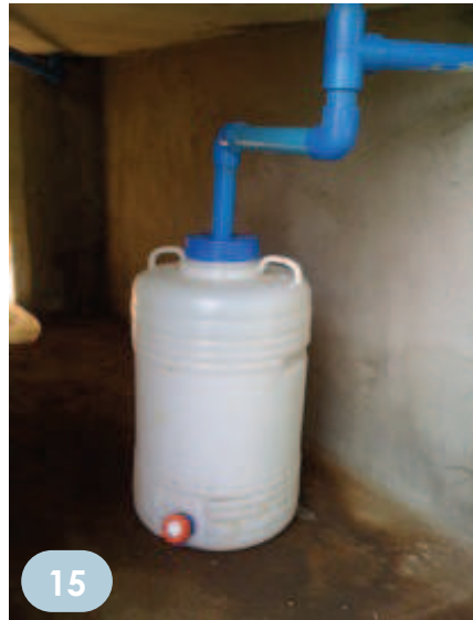
Pic 14: Urine Diversion Dehydration Toilet (Bayawan) Pic 15: Urine collection container of a UDDT (Cagayan de Oro) Pic 16: EcoPee men's urinal for direct urine collection (Libertad)
