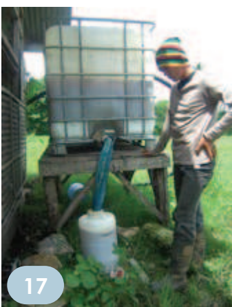
Pic 17/18: Urine Storage in Tanks and Jerricans Pic 19: Transport of Urine from the Households to the Agricultural Production Site (Initao)
