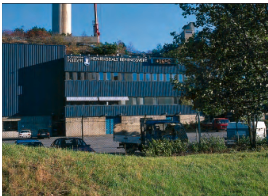
The Henriksdal waterworks in Stockholm ensures state-of-the-art, efficient removal of phosphorus and nitrogen.
