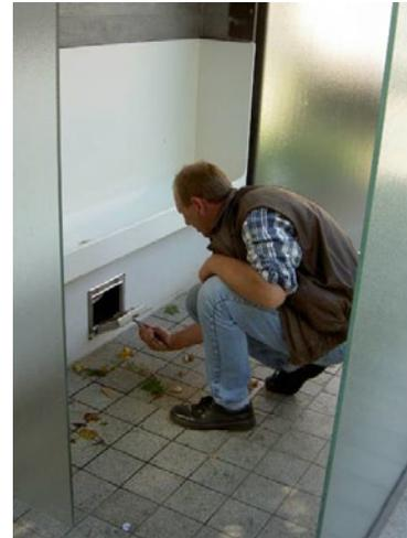
**Fig. 9:** This hatch provides access to a lever to direct urine from the urinal trough either to the sewer or to the urine storage tank (source: P. Grönwall, 2006).
