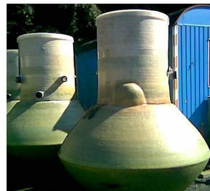
**Fig. 5:** Glassfibre reinforced plastic (GFP) tanks for urine storage before installation (volume 2.5 m<sup>3</sup>). These tanks are buried next to the urinal shed (source: P. Grönwall, 2003).
