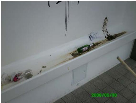
**Fig. 8:** Vandalism and abuse in one of the urinal troughs which led to blockage of the drain pipe (source: P. Grönwall, 2008).
