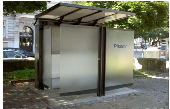
**Fig. 4:** Public urinal shed with waterless urinal trough at Hansaplatz, Hamburg, showing semitransparent walls (source: P. Grönwall, 2003).
