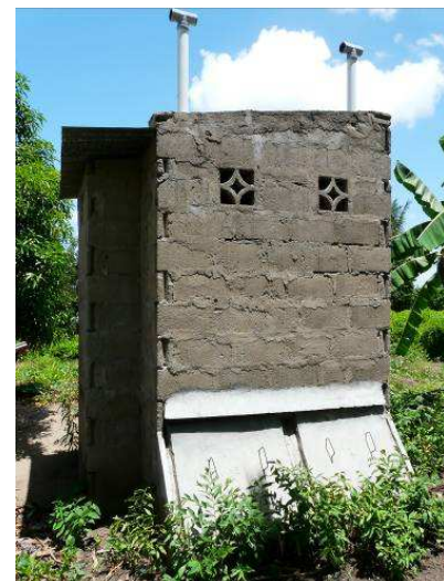
Fig. 12: Household UDDT in good condition, 8 years after construction; note metal faeces vault covers are still in place (source: A. Leitner, 2011).
