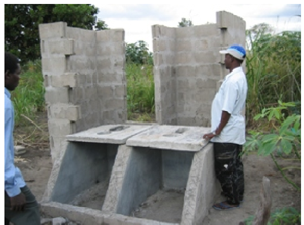
Fig. 4: Construction of a double vault UDDT in 2003; the two faeces vaults are visible at the front (source: M. Fogde, 2003).
