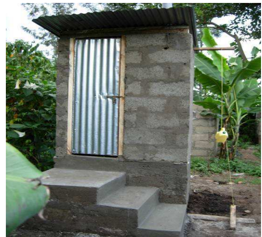
Fig. 5 Single vault UDDTs in Daraja II built with concrete blocks (source: ROSA, 2008).
