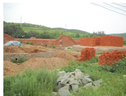
4-in-1 under construction
