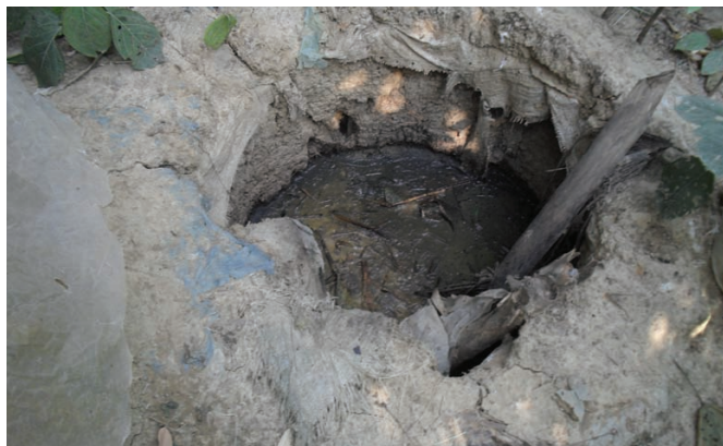
FIGURE 4: OPEN PIT LATRINE IN CHAPAI-NAWABGANJ DISTRICT (CL-3)
