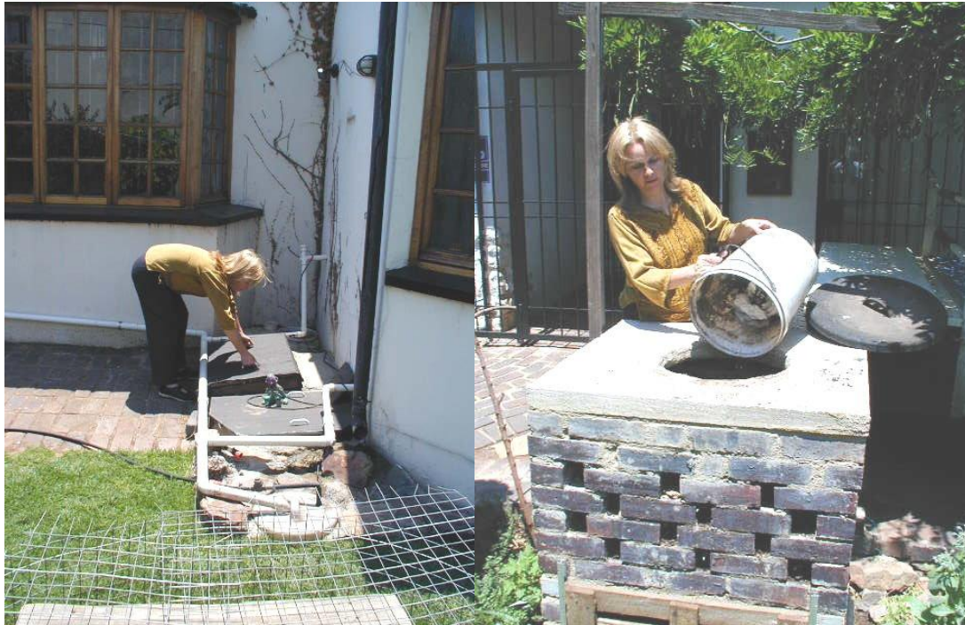
Figure 4: (left) Removing lightweight pit cover, (right) emptying the container into a composter, Johannesburg (source: Holden, 2004)
