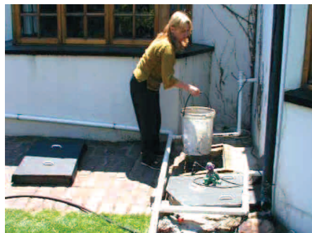
Figure 2: Urine Diversion Toilet with Easily Removable Cover and Emptying of Chamber
