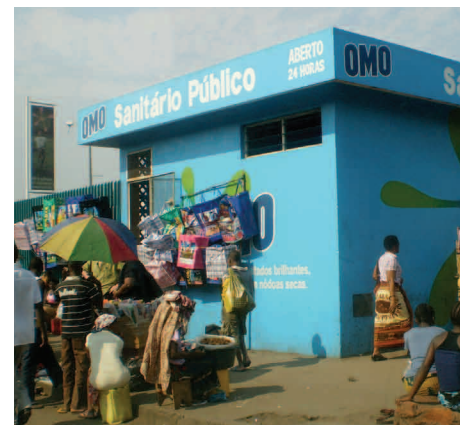
Privately built and operated public toilet in Maputo (© Schaub-Jones)
