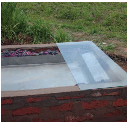
A solar Sludge Drier under Construction
