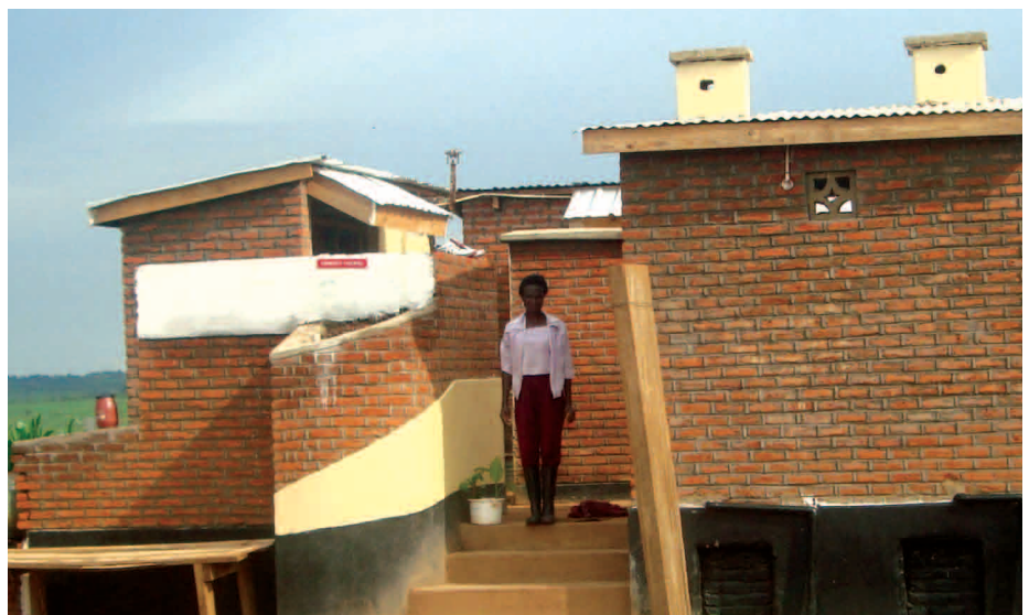
An Ecosan toilet at Chinsapo market
