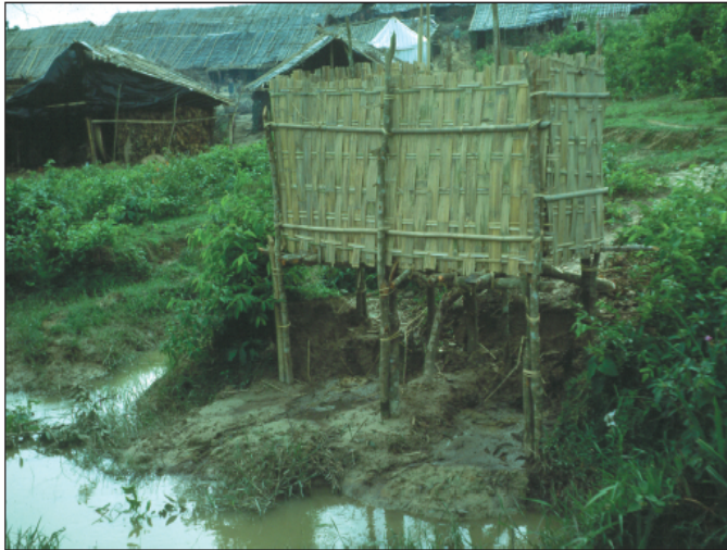
Figure 10-13 Over-hung Latrines Used in Bangladesh (Harvey et al. , 2004)
