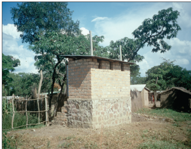
Figure 10-8 An example of a Raised Pit Latrine used in Tanzania (Harvey et al. , 2004)
