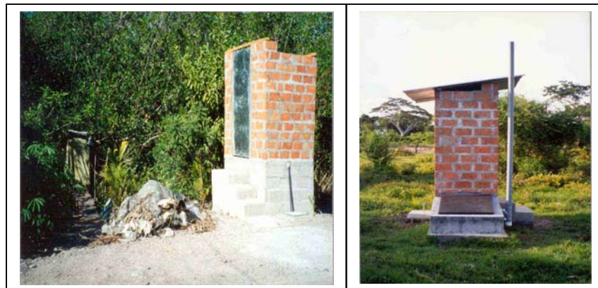
Figure 5-2 LASF Latrines; on the right hand side is the LASF with Solar (Adapted from MSFH Archives)
