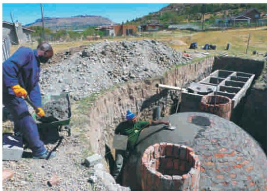
The vertically working Filter Reactor is an optional treatment step, as it is adapted to the Baffled Reactor. Pre-treated water passes through a filter material like stones, gravel or recycled plastic material (bottles). These surfaces are proven to offer living space for bacteria dedicated to absorb organic particles. Like in the Baffled Reactor the water passes the filter vertically from the bottom to the top. The filter reactor can also consist of several chambers.
