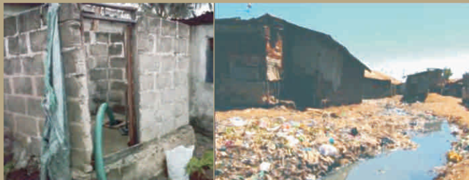
Fig. 4: A typical urban toilet in Tanzania. This needs to be emptied rather than moved. © David Schaub-Jones
