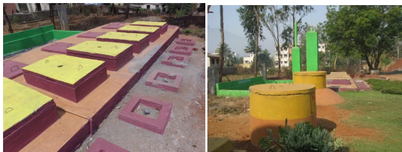
Yellow slabs of the ABR Chambers The circular neck chamber of BS
