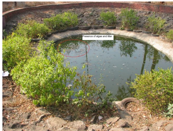
Presence of algae in the polishing pond
