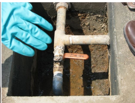
Water trap inside a chamber
