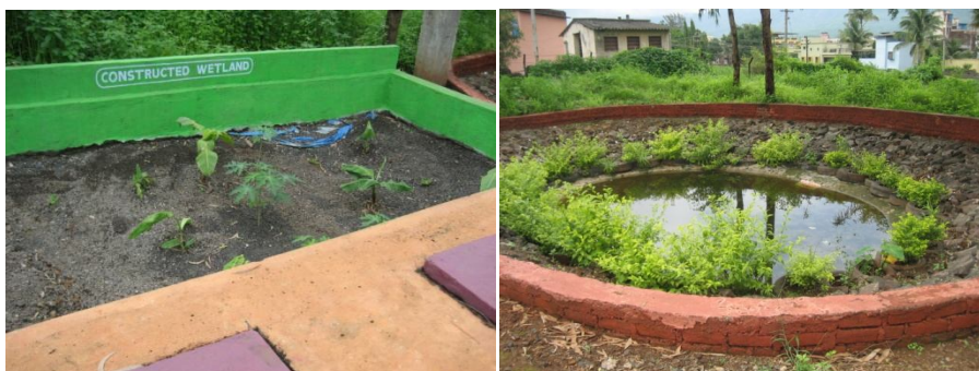
Planted Gravel Filter
