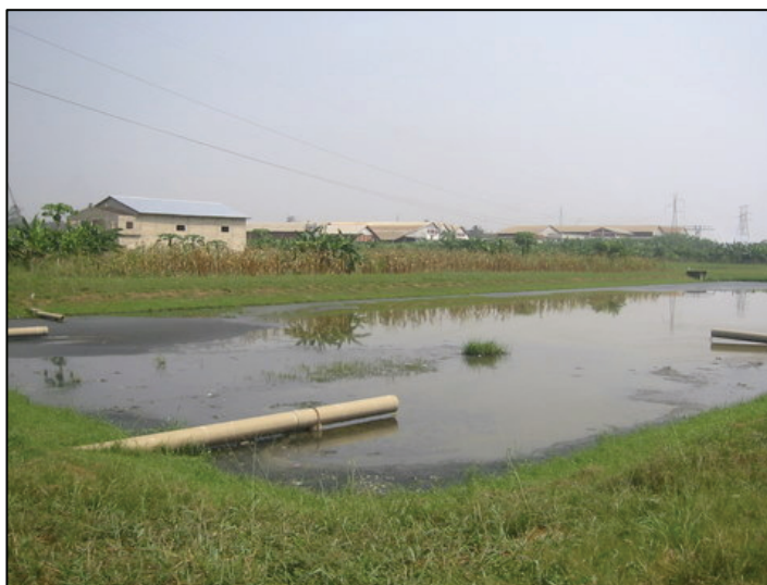
Figure 3. Sedimentation pond at Asafo, Kumasi
