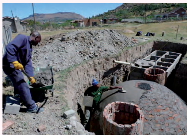
Figure 3: Approaching the final stage of construction: biogas digester and anaerobic baffled reactor before being covered with soil and installation of planted gravel filter will start
