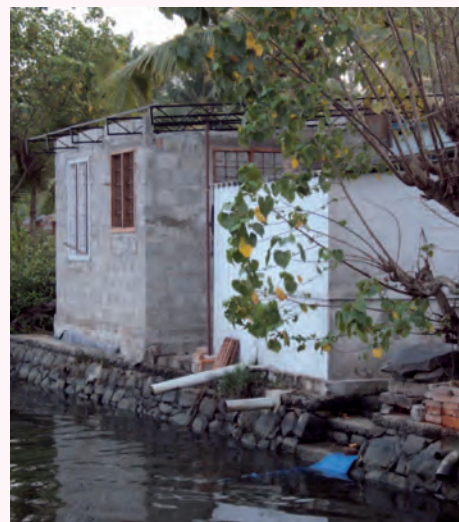
Figure 2: Toilet discharging into the backwaters
