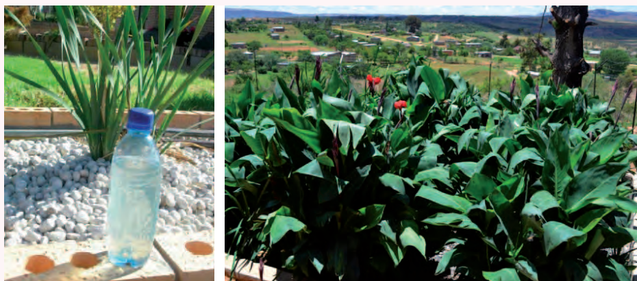
Figure 6: Nice-looking on-site wastewater treatment: treated water at a PGF with recycled pumice stones shortly after system start (left) and PGF after 3 years of operation
