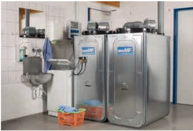
Figure 5: MBR system, (MF-HKA 4, capacity 48 l/h) Busse Inc., Leipzig
