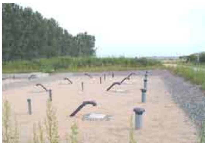
Figure 6: First stage bed just after completion and before reed planting (Photo: Liénard, 2003)
