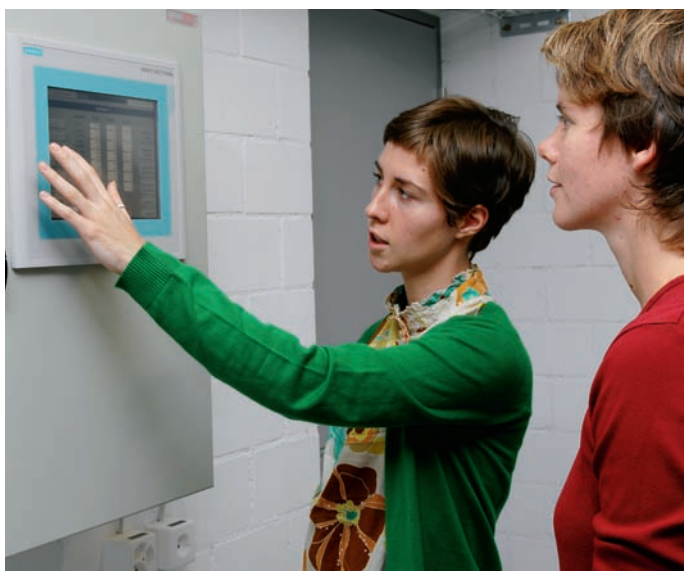
Gone but not forgotten: The date and time of each flush are recorded by a digital counter at Eawag (Photo Ruedi Keller)
