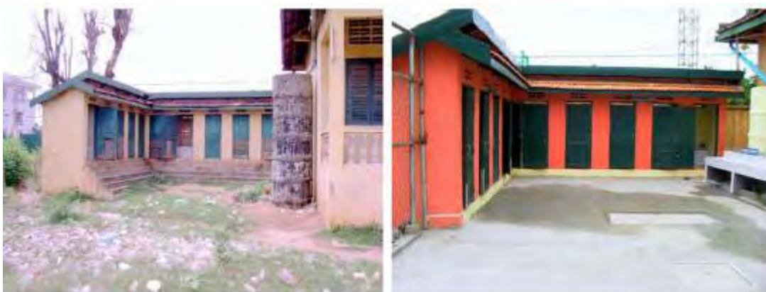
Figure 3. Before and after of the school toilets and new DEWATS at the Chroy Chang Va Primary School project
