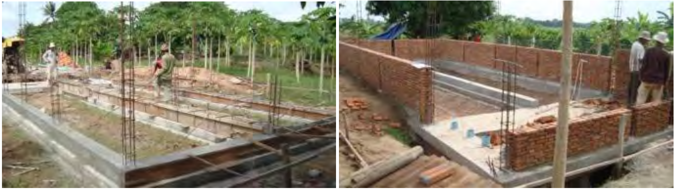
Figure 6. Photos of the plant under construction
