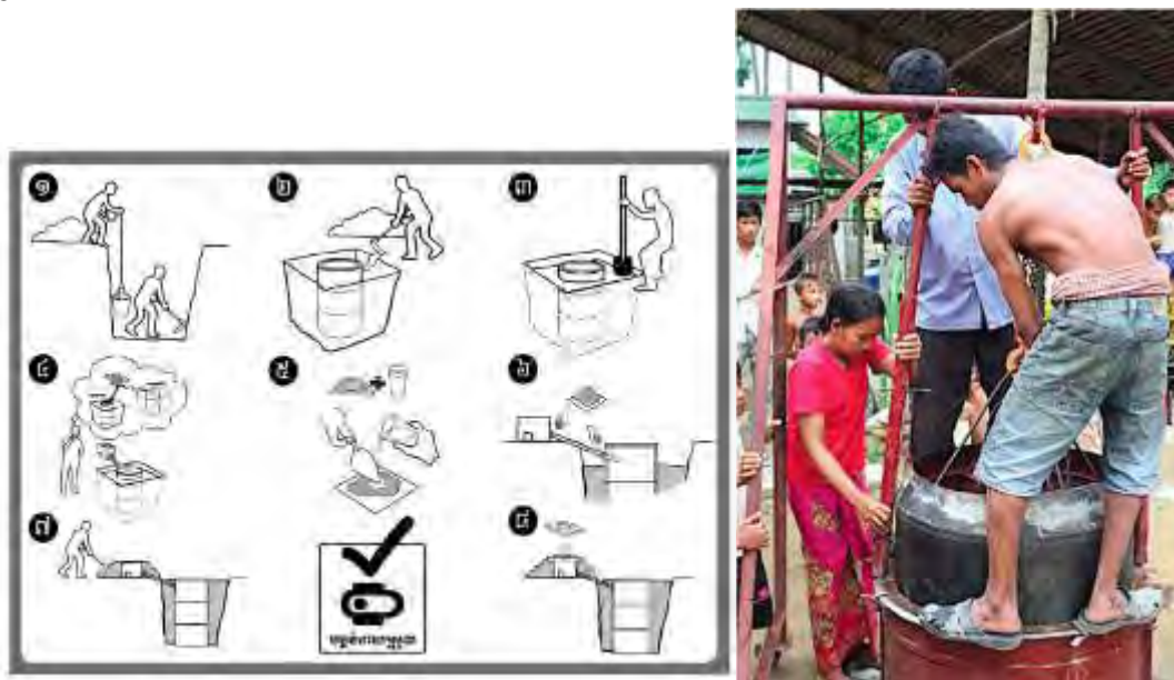
Figure 2. An excerpt from a Latrine Building Manual created by IDE for the businesses (left) and one of the businesses constructing a concrete ring for the pit using their pre-purchased mold (right)
