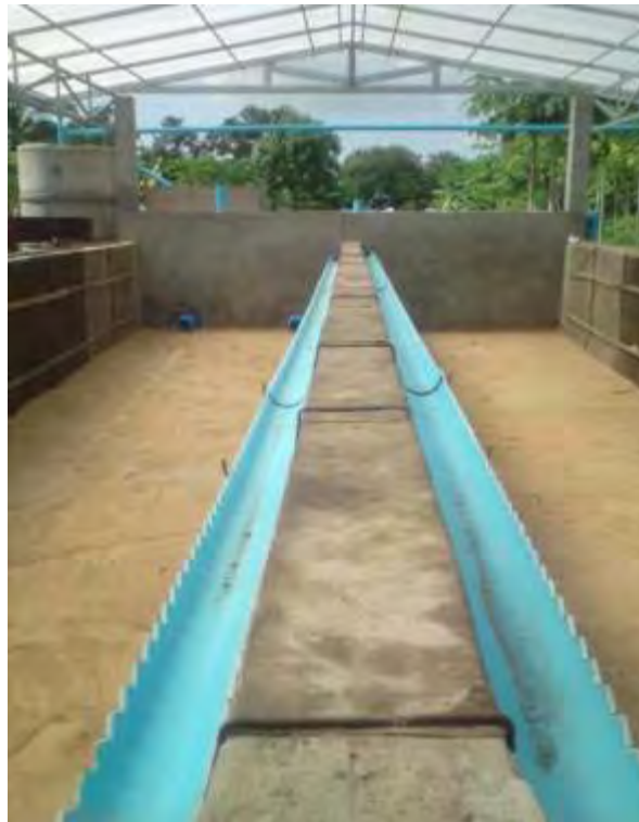
Figure 7. Photo of the SDBs and their inlet troughs, also showing the two drainage valves from the solid extraction settler and the aerobic pond
