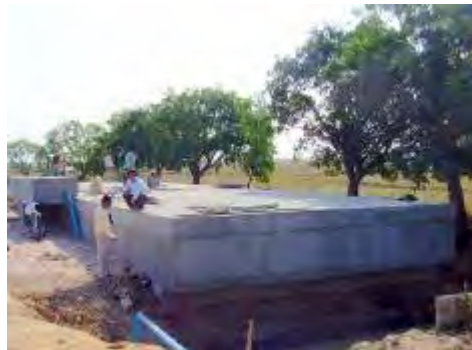
Figure 2. Construction underway at the Trapeang Sab Commune project
