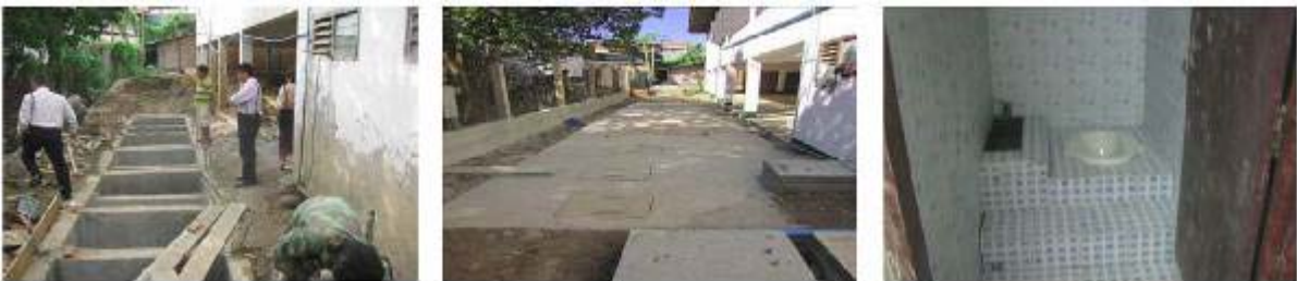
Figure 3. Construction and renovated toilets at the Khoualuang Primary School project
