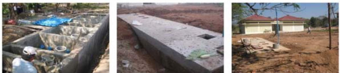
Figure 4. Construction and completed works at the AFC project
