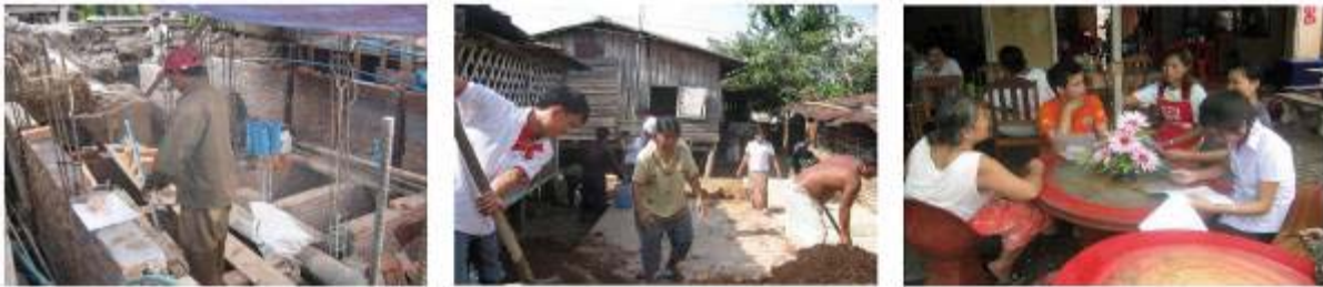
Figure 2. Construction and community engagement at the Thongkankham Village project
