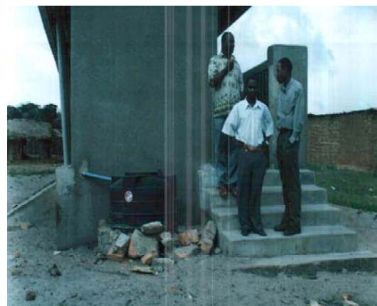
Figure 3: The newly built Ecosan toilet for the shoreline fisher village in Dimo Rakai District, Uganda. In the fore is the urine container.
