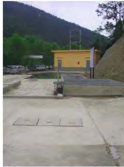
Figure 2. Photos of the bear rescue center’s DEWATS under construction and completed
