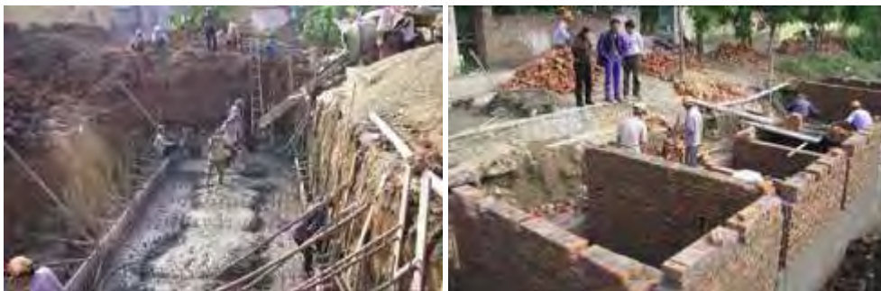
Figure 2. Photos of the DEWATS under construction
