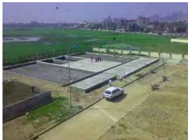
Figure 5. Photo of the completed HGF of the Kim Bang District Hospital project
