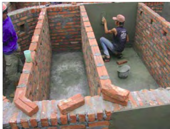
Figure 2. Photos of the private home's DEWATS under construction
