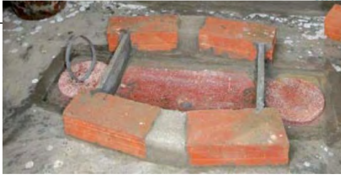
Figure 2: An example of an installed Granito pan with 2 covered defecation holes (Photo courtesy of PLAN Vietnam)
