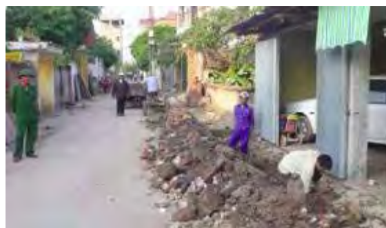
Figure 3. The gravity-fed sewer line under construction
