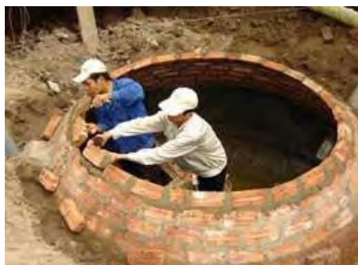
Figure 4. A biogas digester under construction by one of the program BCTs
