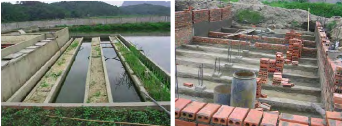
Figure 2. Photos of the slaughterhouse DEWATS under construction
