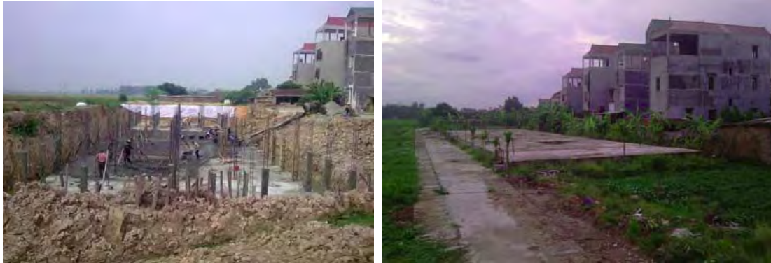
Figure 2. Photos of the commune DEWATS under construction and completed
